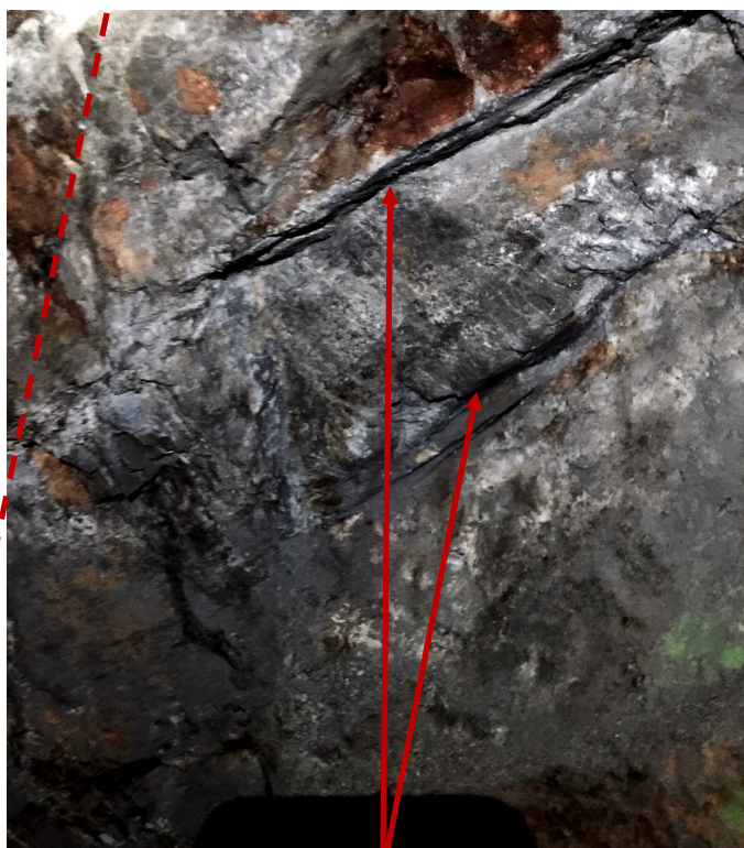
The veinlets on the face have had 6" of material removed. The veins of Mo are extensive. Tunnel #3
